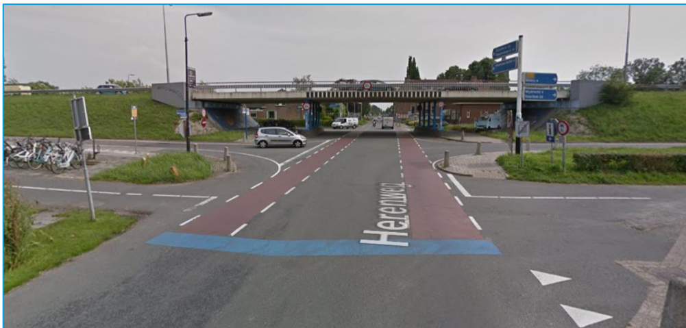
Herenweg, viaduct N201. Bron: Google Streetview
